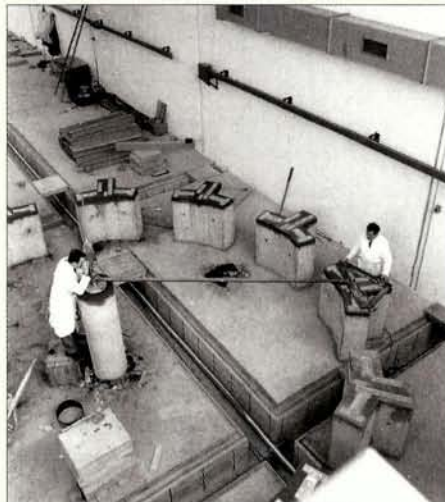
"One of these possibilities...is the construction of so-called 'storage rings'." J Brüderlein (left), from PS Survey Group, and W Sax, Engineering Drawing Office, are here engaged on levelling the foundation supports for a storage-ring model being built by the Accelerator Research Division.
