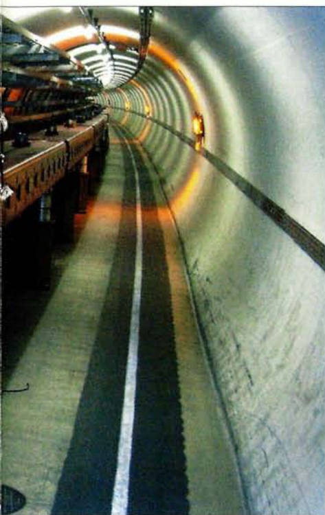
a corrector (green) and a series of main dipole magnets installed in the LHC tunnel in Novosibirsk, Russia.
